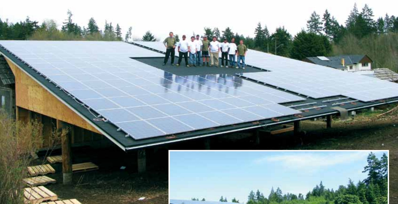
T'Sou-ke Trainees completing 40kW Photovoltaic System.
